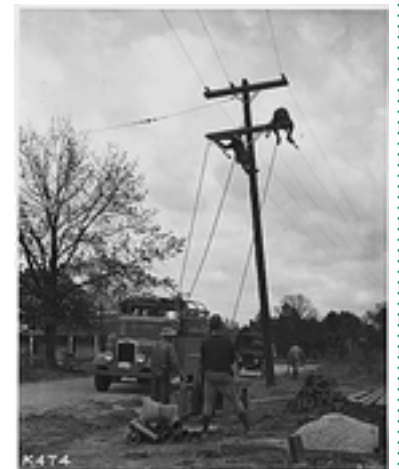
REA installs power lines, 1936.
