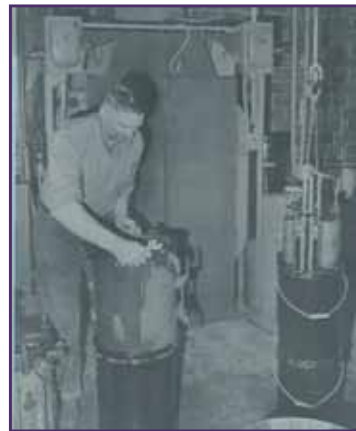
Frank recoring a transformer in 1966
