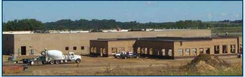
People's Cooperative Services new headquarters building under construction.
