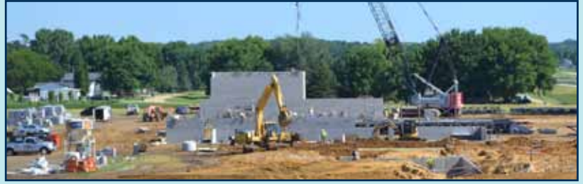
People's Cooperative Services new headquarters building.
