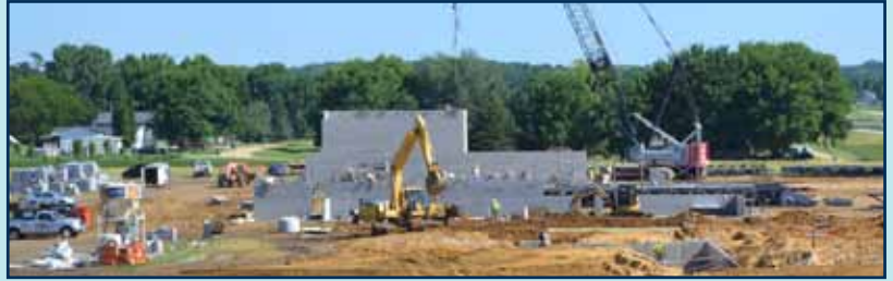
People's Cooperative Services new headquarters building.
