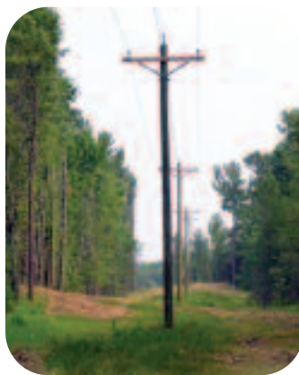
Right-of-way after clearing.
